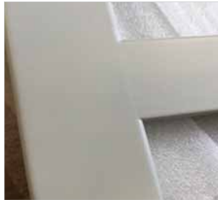
Slight step in the joint between frame and rail. Paint unbroken.
